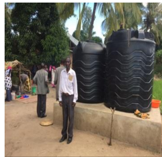
Dihombo Water Purification
