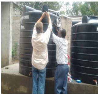
Temeke Water purification
